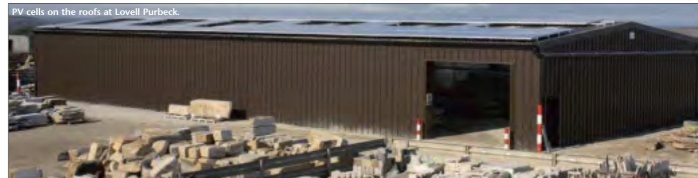
PV cells on the roofs at Lovell Purbeck.
