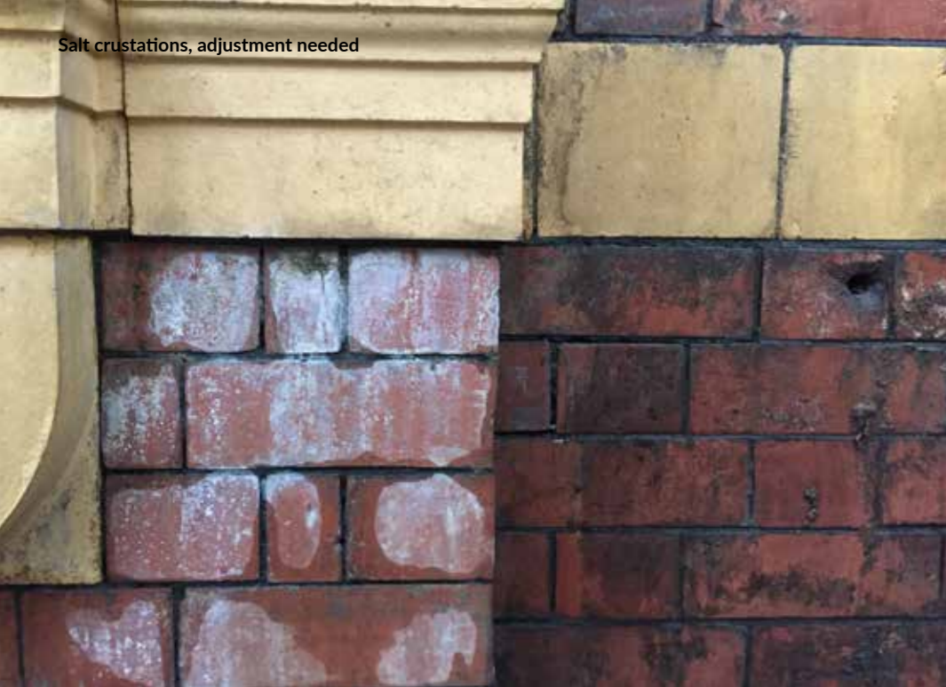
Test sample clean on terracotta
