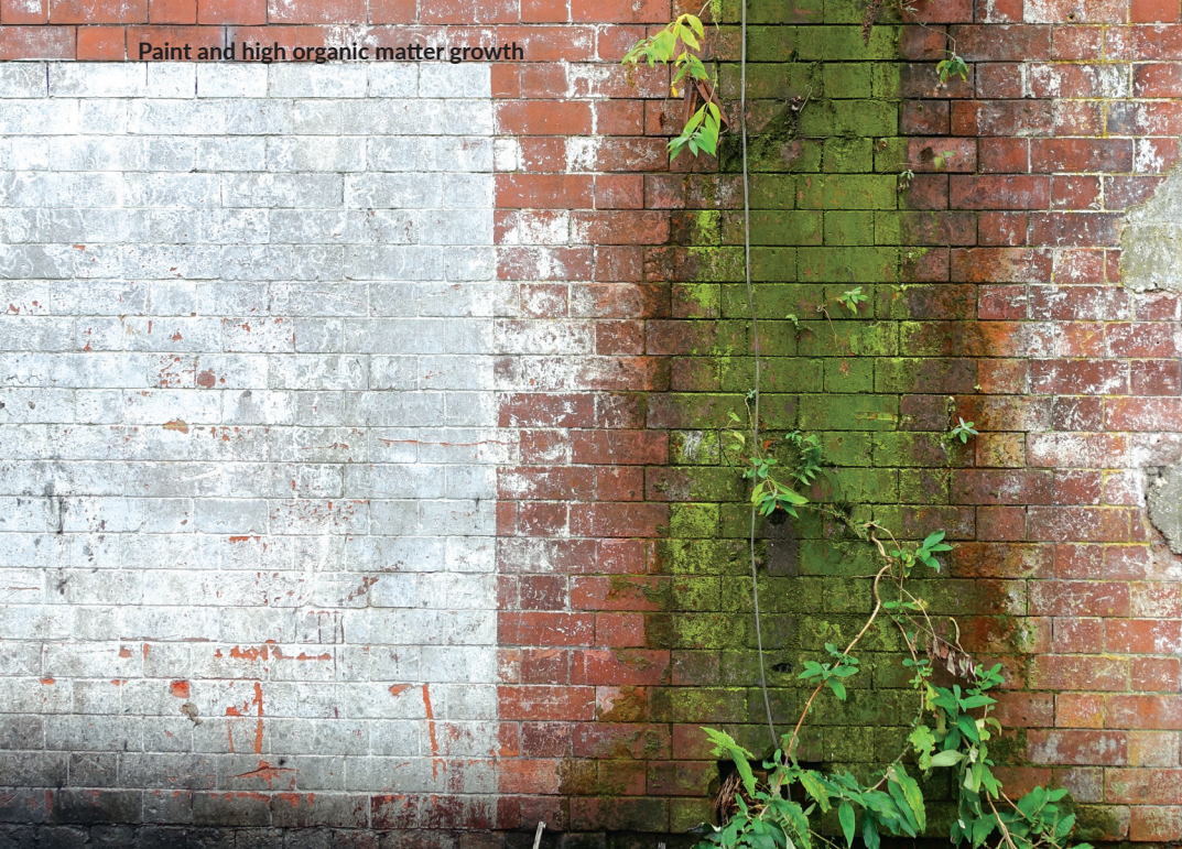
Loose paint and brick façade
