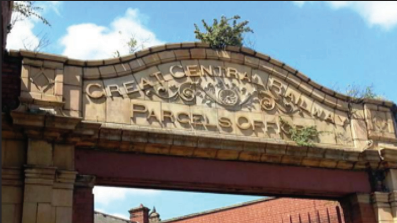
Large ornate terracotta archway leading to the main gateway to the former
