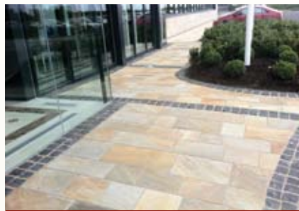
▲ Paving & Limestone Setts
