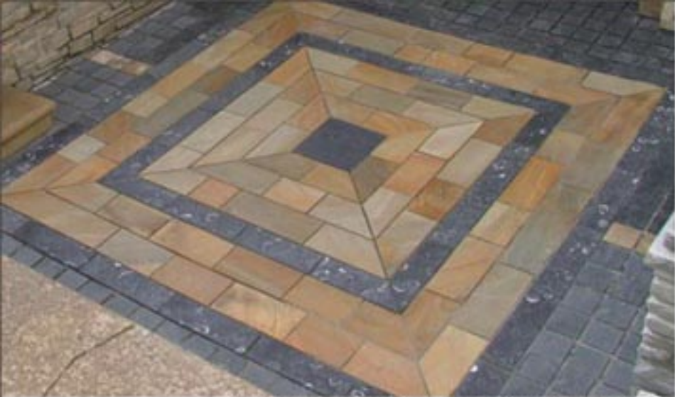
Celtic Square – Donegal Quartzite Tiles & Irish Limestone Paving
