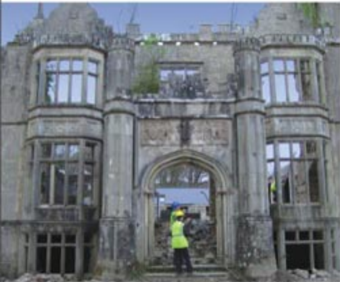
Castle Prior to Restoration
