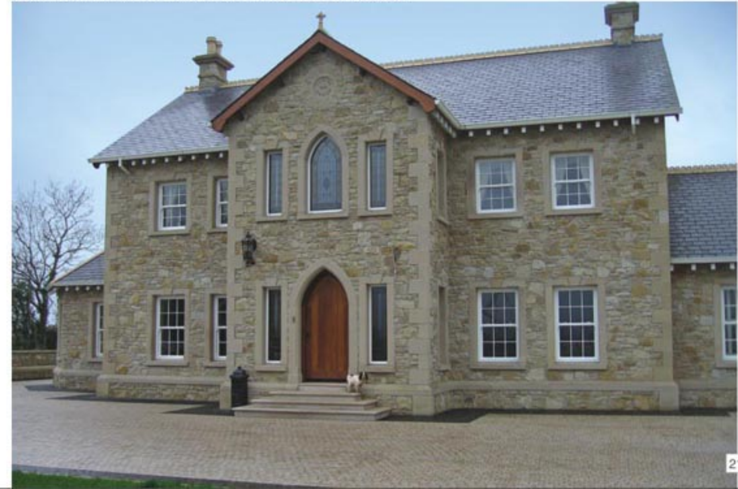
Brown Random Rubble with Sandstone Quoins, Plinth, Door and Window Surrounds
