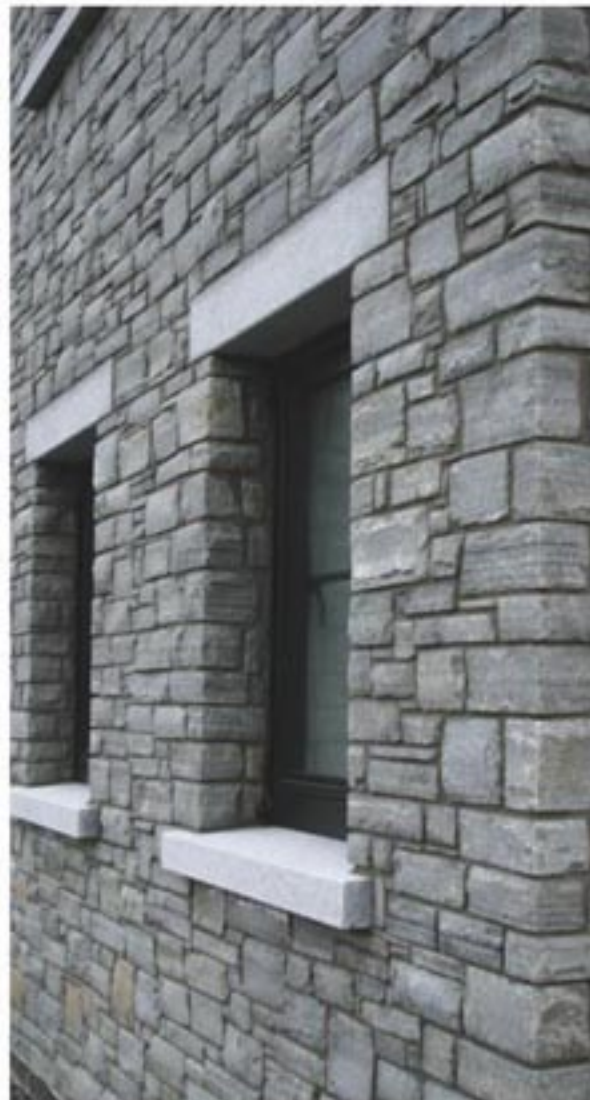
Grey Machined Block with Silver Granite Cills & Lintels
