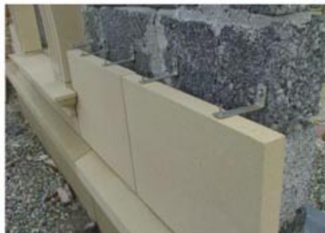
Fixing of Ashlar Cladding
