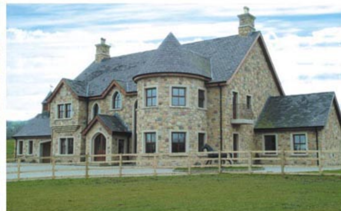
Mixed Random Rubble with Sandstone Door and Window Surrounds
