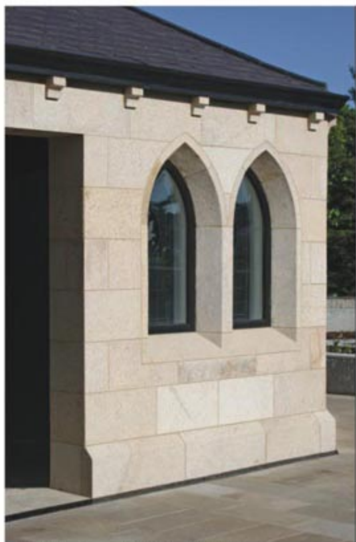
Gothic Window Surrounds, Cladding, Plinth & Paving
