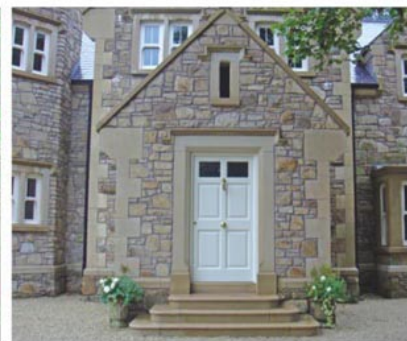
Door Surround, with Moulded hood, Quoins & Kneeler Stones to Support Barge Coping
