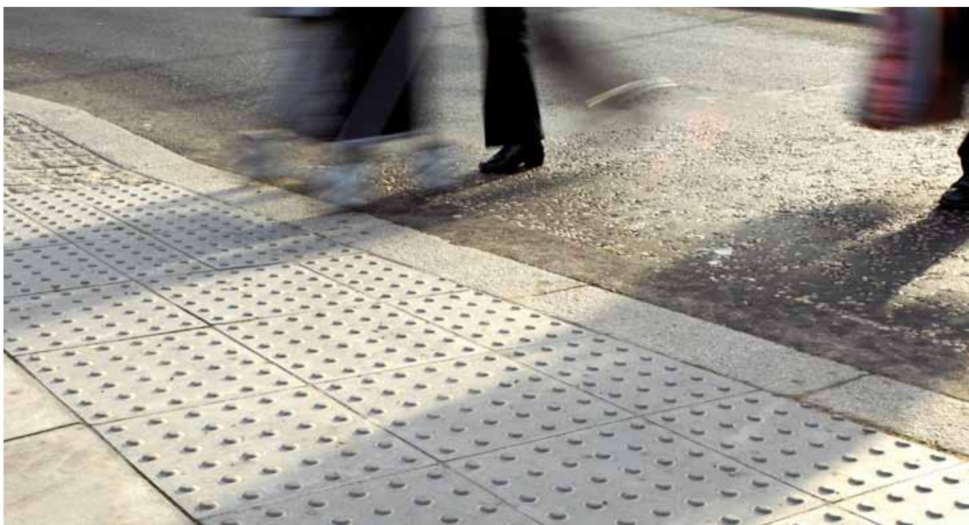
Blister Tactile Paving
