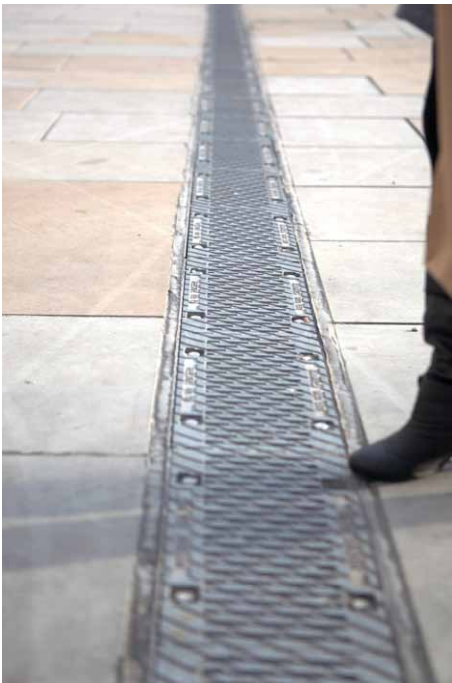
Elizabethan Mix Sandstone and Birco Drainage
