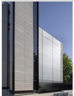
To ensure they specified a stone in harmony with the existing Grade 1 listed building, it was important for RSH+P's design team to understand the stone's physical characteristics and it's performance on several historic buildings. To help with the selection process we arranged a guided City and West End Tour to show them different beds of Portland stone on several historic and contemporary buildings.
