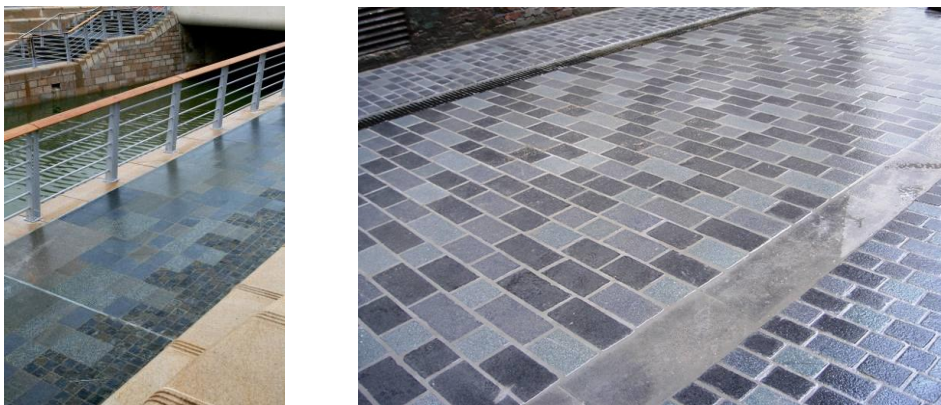
Fig 1. Rich mixes created with a variety of granites at Pier Head & Cavern quarter, Liverpool.
