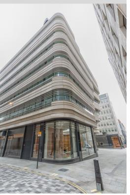
The second block, adjacent to Haymarket, is open jointed. It involves a curved Portland Stone and glass wall wrapped around the building using 3,400m<sup>2</sup> of Jordans Whitbed on a unitized facade with horizontal aluminium fins.
