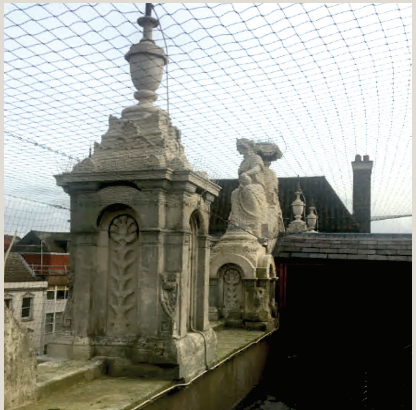
Works in progress
