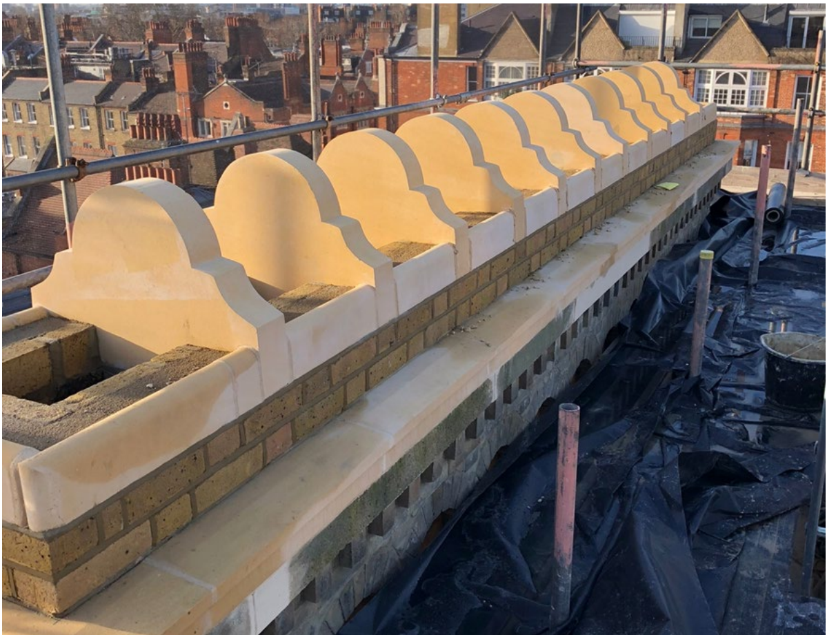
Newly constructed top section of stack, using reconstituted Bath Stone and new yellow stock bricks.
