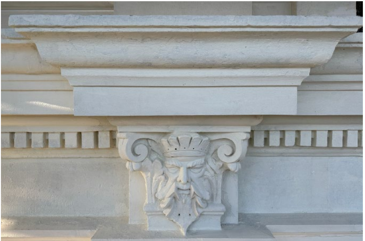
Completed Bath Stone repairs and redecoration.
