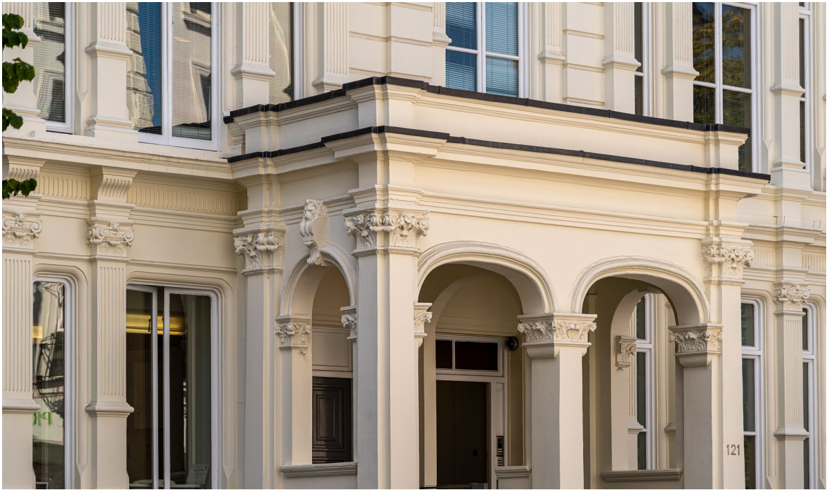
Completed: New Lead Capping's to Restored Portico
