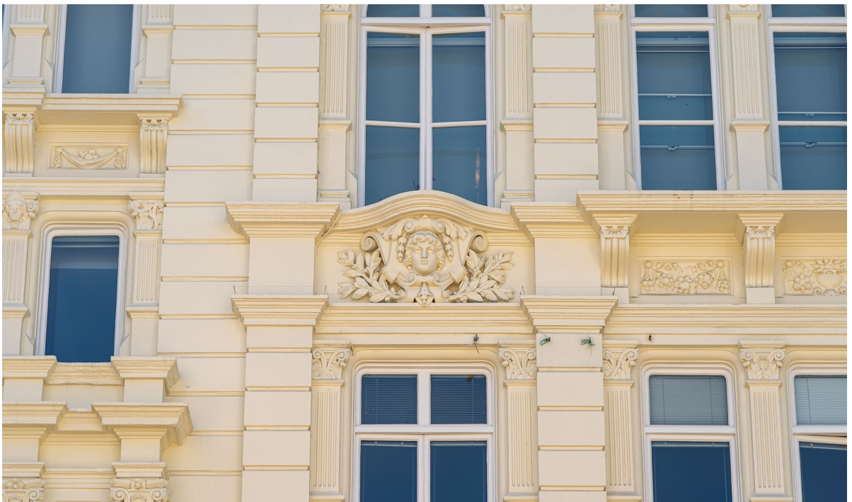
Completed: Restored Ornate Bath stone Gargoyle
