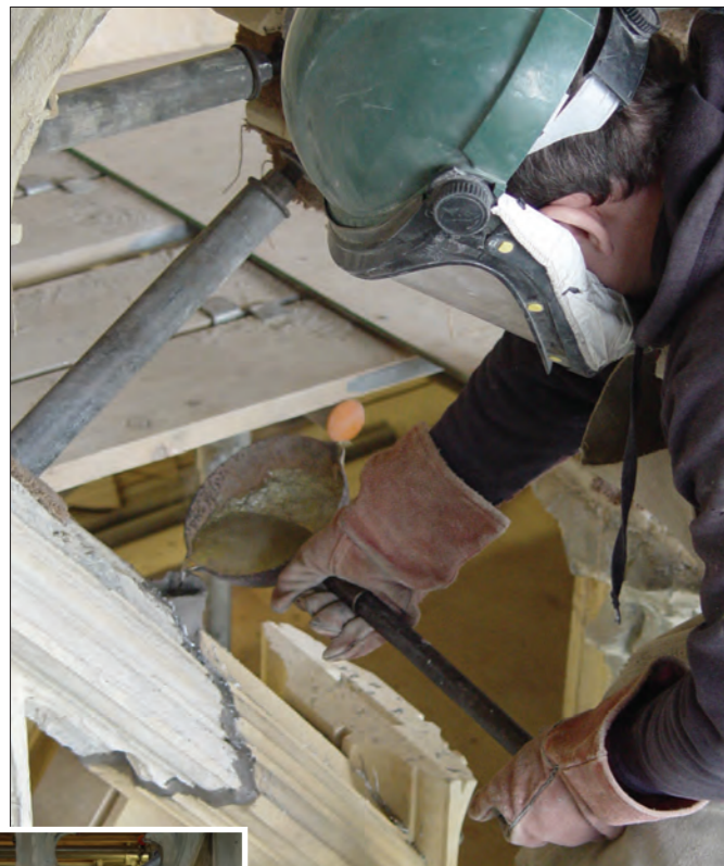
Above. The masons at the Minster have learnt from their predecessors and are using molten lead to create the joints between the stones of the tracery on the Great East Window. This is Lindsay Hogarth pouring the lead.
