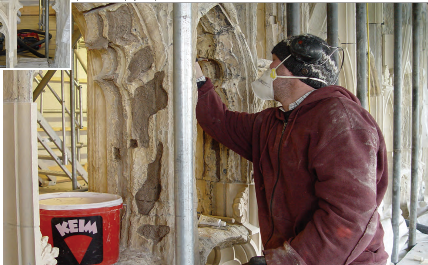
Below. Keim fillers are being used to repair the stone where it is still structurally sound. Nanolimes are also being used. John Sutcliffe is pictured here carrying out repairs.
