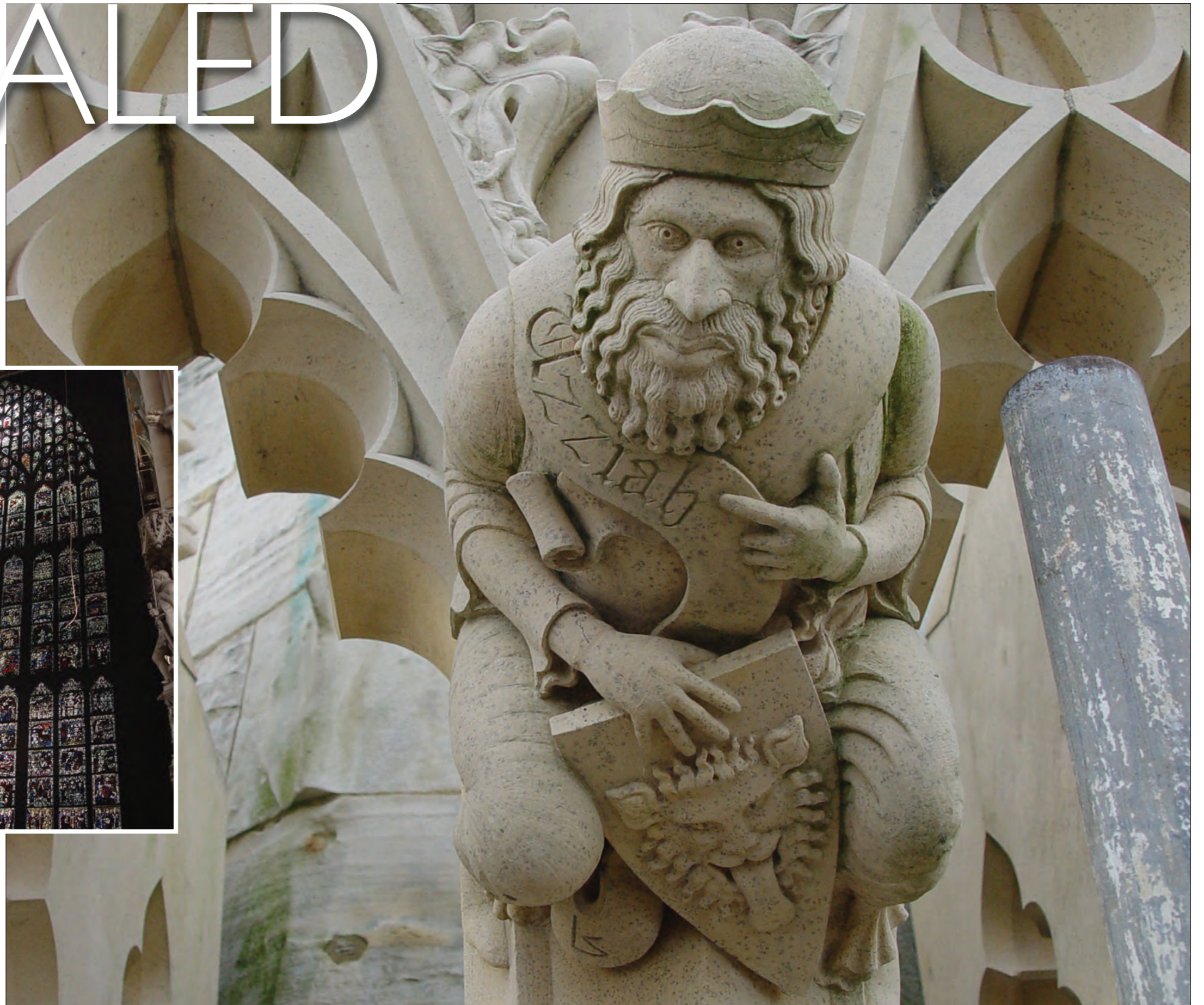
Right. One of the carvings and new masonry on the rebuilt southern buttress of the East Face of the Minster that gained the Minster's masons top honours in the Craftsmanship category of the Natural Stone Awards in November.
